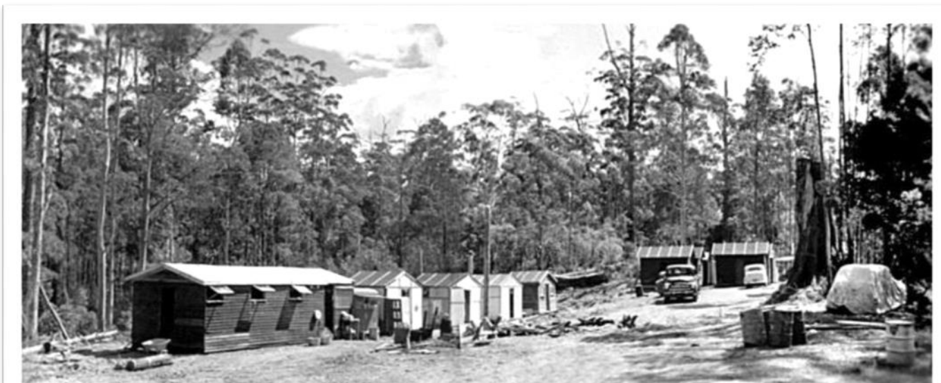
The Cape Horn road construction camp on the Great Ocean Road, north of Apollo Bay.
