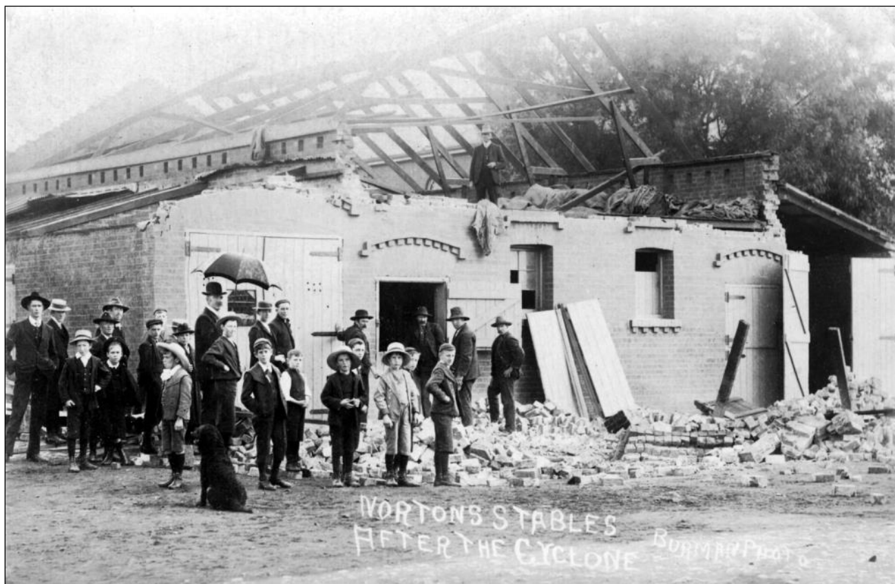
Norton's stables after the cyclone, photo by A.W. Burman This building is now occupied by Cinnamon restaurant in Wood Street. EGHS collection
