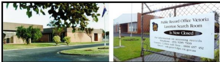
The Laverton building
