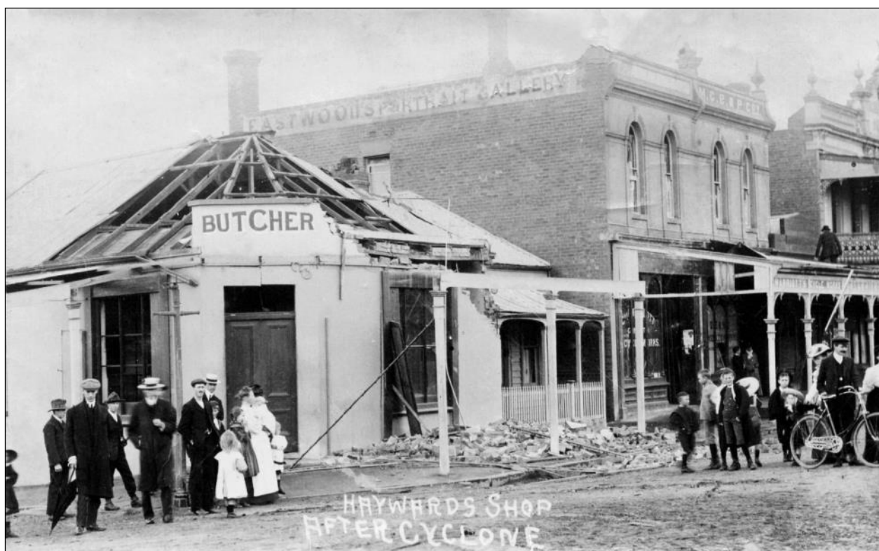
Hayward's Butchers shop wrecked; also Marriot's roof carried away during cyclone. These buildings were on the south west corner of Main/Wood Street. EGHS collection
